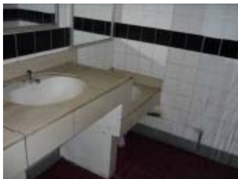
Photo 4-1-3 Accessible toilet at Kelana Jaya Station
