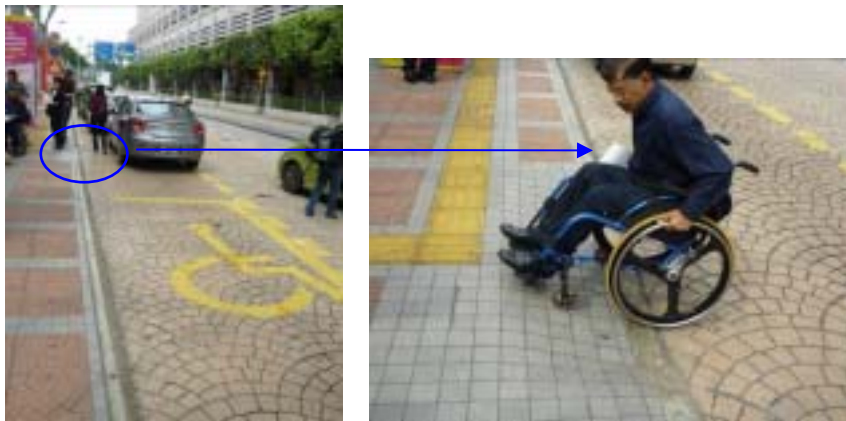
Photo 4-1-2 Access to sidewalk from accessible parking
