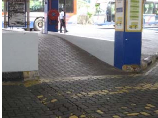
photo 2-5-9 Bus terminal slope (Kelana Jaya)
